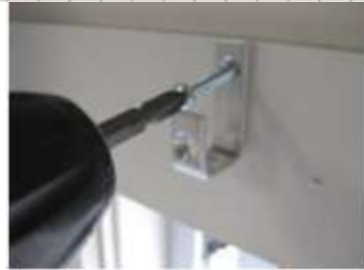
Fig.2 Face mounted using long screw
